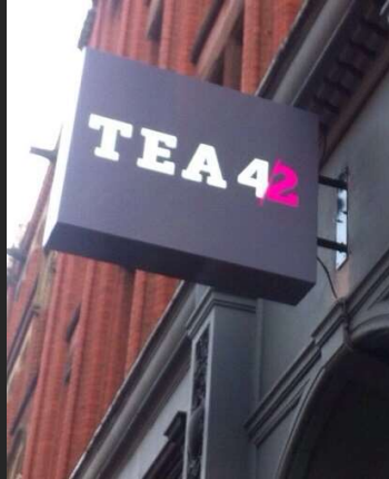
Fixed projecting boxed sign that can be 'fret-cut' & illuminated from within as seen on right
